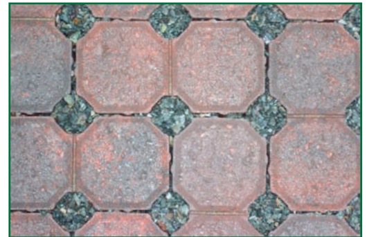
Joints between pavers are filled with small stones to provide permeability
